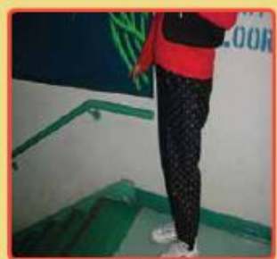
Figure 7.1. Handrail was lowered in order to hang large picture above; handrail too low to be of use
