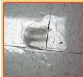
Figure 3.2. Dented vinyl tiles
