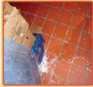
Figure 1.2. Water on floor caused by pipe splashing water.
